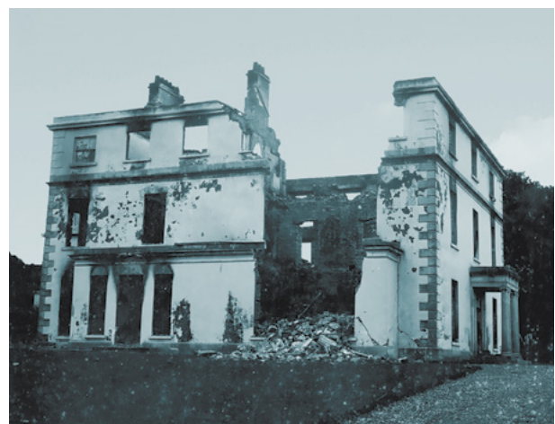
Kiltannon House in Co Clare, burned on 3 September 1920.
