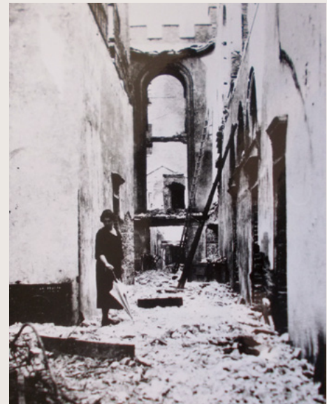
Mary Gaussen, niece of Lord Bandon, going through the ruins of Castle Bernard. Co Cork. IRISH ARCHITECTURAL ARCHIVE
